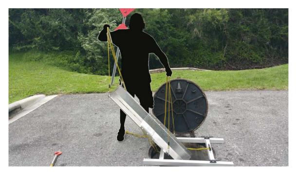
6. The platform is in place when the tongue is inside the invert and the body of the platform is even with the outside lip of the invert as shown below. If the invert cannot be reached, you can extend the length of the platform and move the front ropes further back to gain some additional distance. During this procedure, the front ropes are used mostly for guidance, while the rear ropes and tongue provide platform support.
