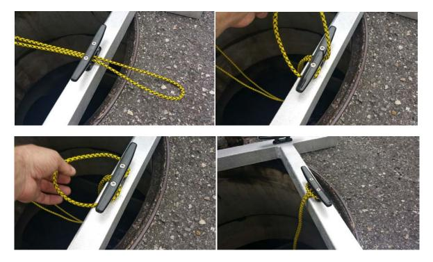
5. Gather the rear ropes in one hand and the front ropes in the other. Angle the front of the platform into the pipe and lower the assembly while guiding the tongue of the platform towards the lip of the invert.
